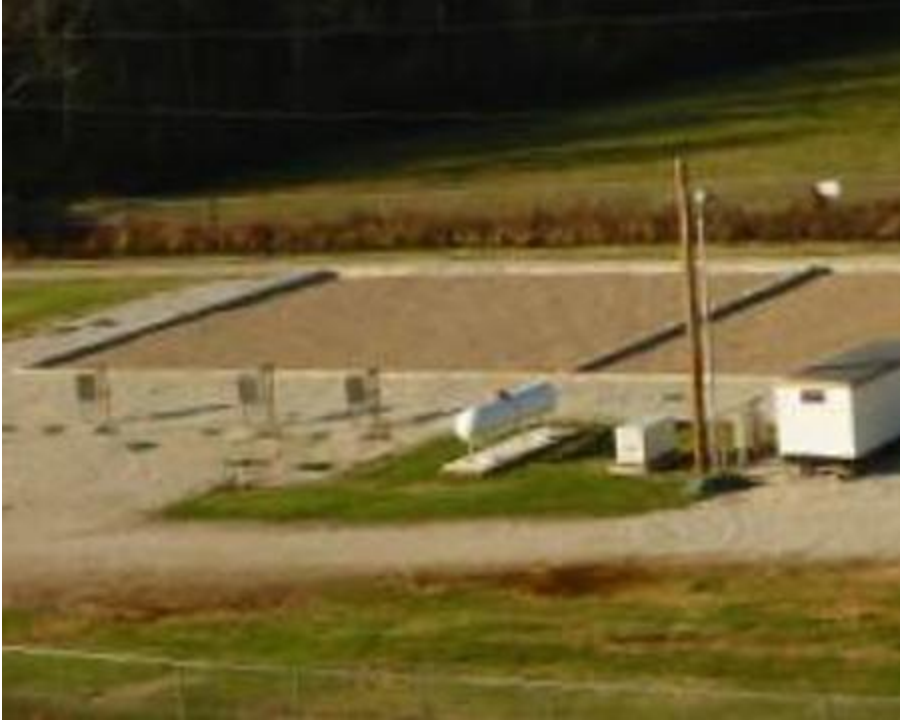
PWSD#13 wastewater treatment plant
